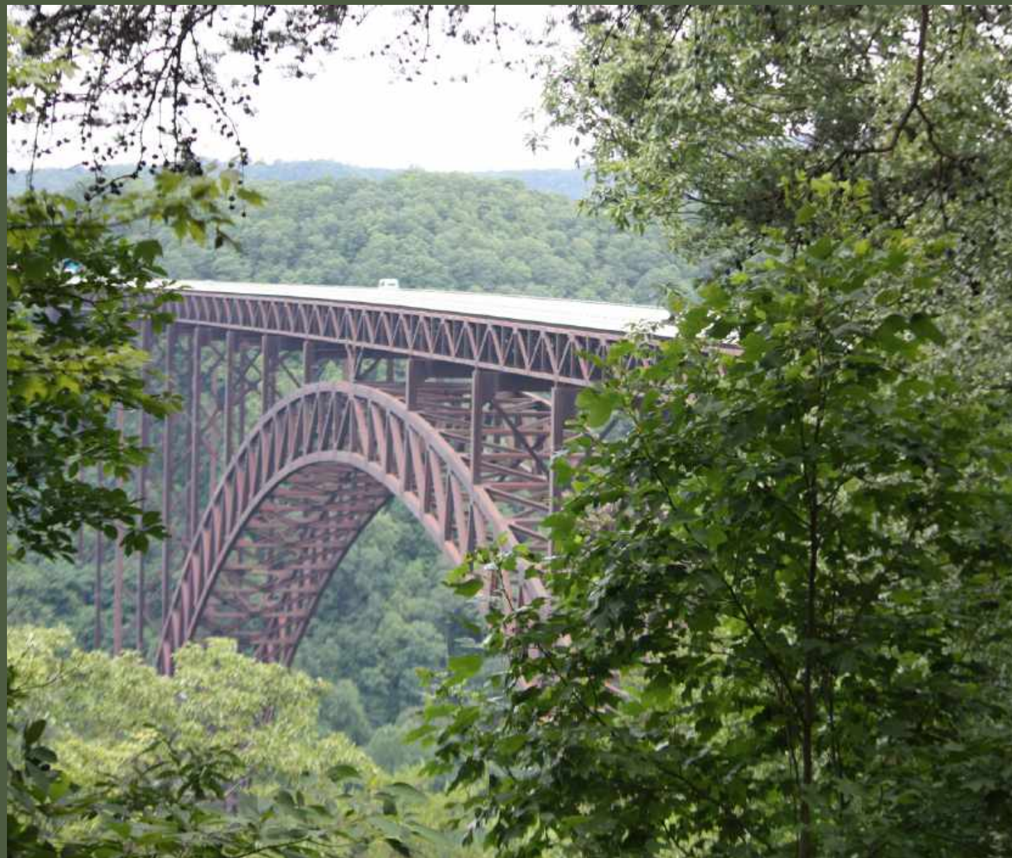
Photo taken of New River Gorge Bridge in Fayette County, West Virginia.
